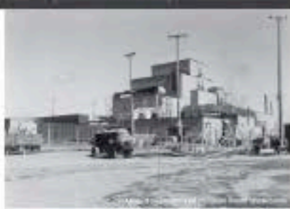
Construction of Hanford's B Reactor, the world's first full-scale plutonium production reactor
