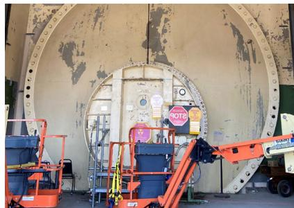
TMI-2 Reactor building equipment hatch
