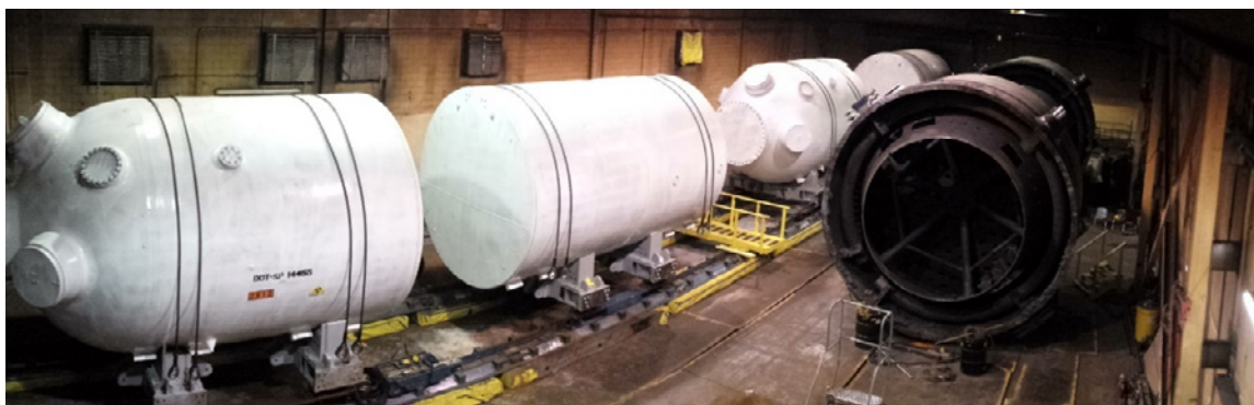
St. Lucie steam generators in “D Shop” of E Building
