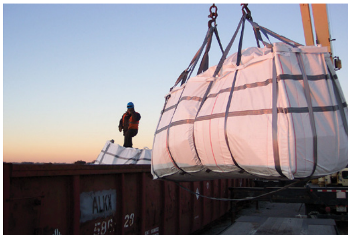
FLEXIBLE WASTEPACK BEING LOWERED INTO A RAILCAR
