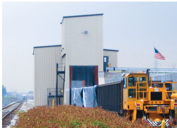
TRACK MOBILE POSITIONING LINED GONDOLA RAILCARS AT MHF FACILITY
