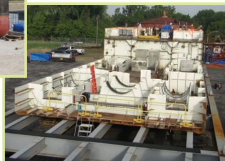
Segmentation halfway complete; work platform visible in foreground
