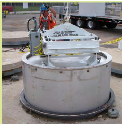
Final disposition into in-ground containers
