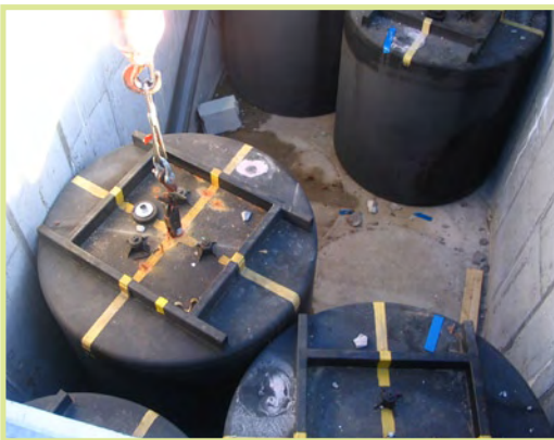
Retrieval operations from storage trench
